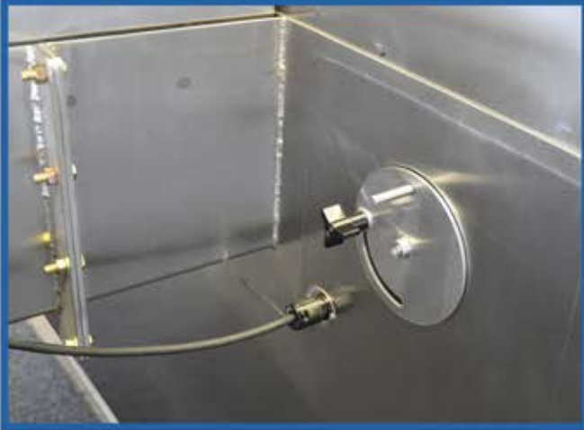
Butterfly air flow control valve.
